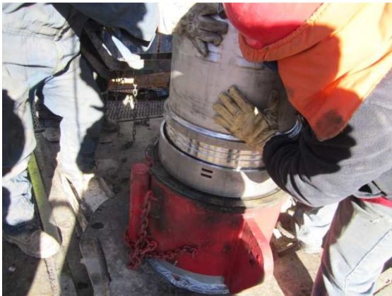
#4 Male and female ends are joined
