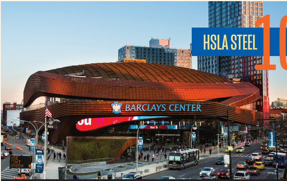
Barclay's Center in Brooklyn, NY. Exterior façade constructed from HSLA Steel.
