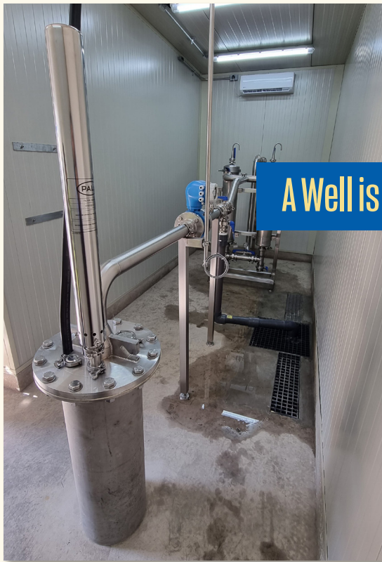
Pump House and Completed Well Head
