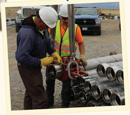
In the spring of 2021, Idaho National Laboratory, **Case Study** which is operated by **Battelle Energy Alliance** for the **Department of Energy**, required stainless steel 304L pump column for its well located in eastern Idaho. **American Pump**, based in Idaho Falls, contacted Roscoe Moss Company after learning about the unique double spline lock couplings that can be used on either well casing or pump column.
